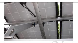
Side Solar Array: unlok pins, position Solar Module and Pin.
